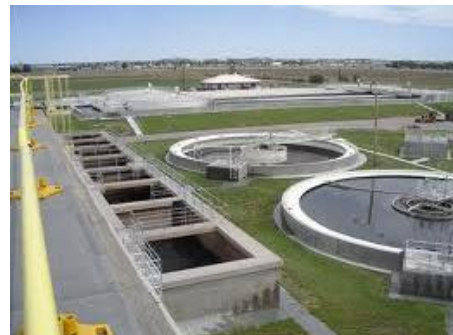
City Waste Water
