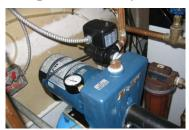
The WEPS14 is a wireless pressure sensor that can measure up to pressures of 15,000PSI, so it is ideal for Hydraulic Pump applications. For monitoring , the WEPS14 offers temporary remote Pressure measurement of the system. The battery powered solution can last up to 24-months of continuous (1 measurement/30 seconds) use.
