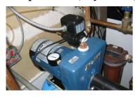
The WEPS04 is a wireless pressure sensor that can measure up to pressures of 15,000PSI, so it is ideal for Hydraulic Pump applications. For monitoring, the WEPS04 offers temporary remote Pressure measurement of the system. The battery powered solution can last up to 24-months of continuous (1 measurement/30 seconds) use.
